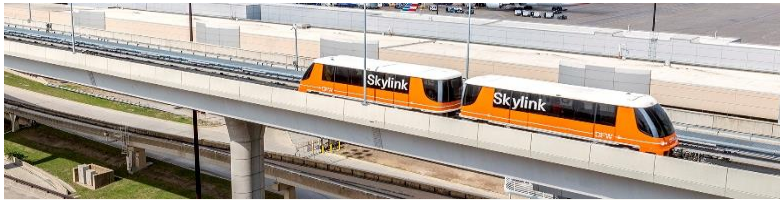
DALLAS (10 YEARS OPERATION & MAINTENANCE – US)
